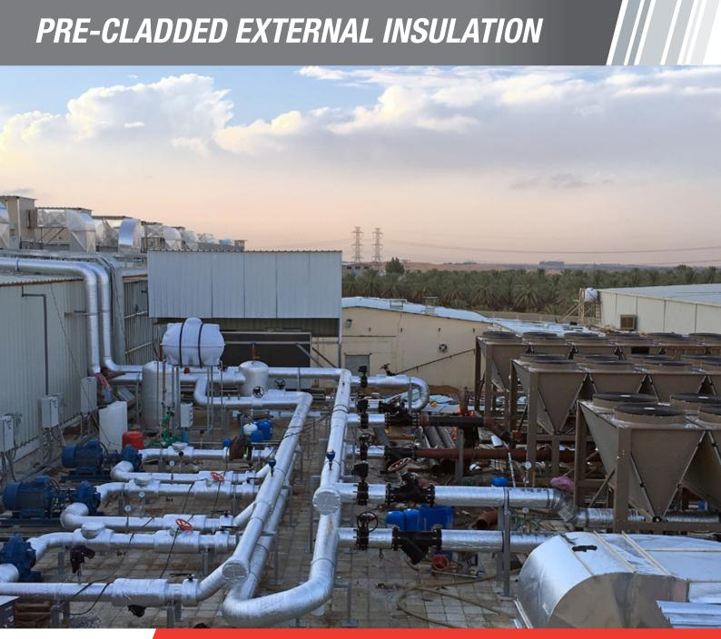
Closed cell, physically crosslinked polyolefin foam insulation with innovative ultra tough foil facing for external applications.
