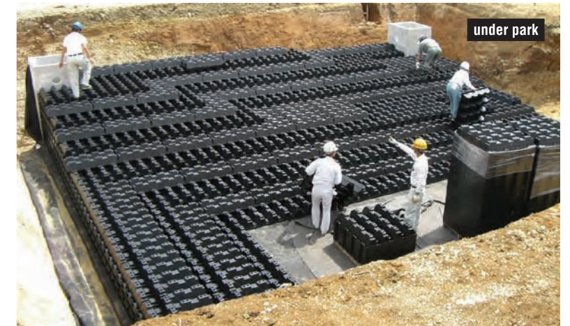
Rainwater regulating reservoir in Chiba prefecture at group housing society (storage capacity:420m 3 )
