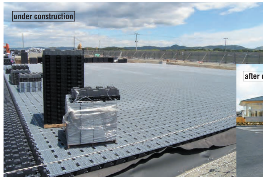
Rainwater regulating reservoir construction for government office in Miyagi prefecture (Storage capacity:1,700m 3 )
