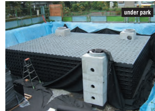
Reservoir construction in Tokyo for rainwater utilization (Storage capacity:100m 3 )
