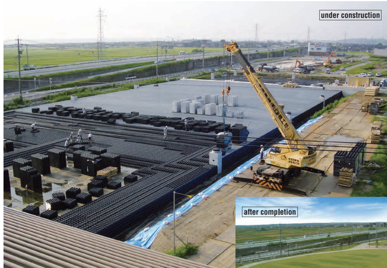
Rainwater regulating reservoir construction in Ishikawa prefecture (Storage capacity:9,200m 3 )
