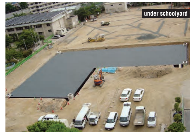
Rainwater regulating reservoir construction in Fukuoka prefecture under playground at school (storage capacity:800m 3 )
