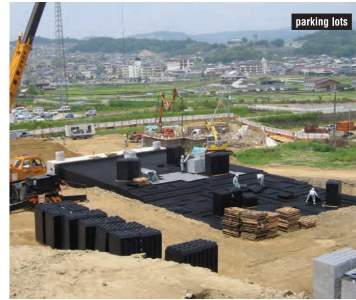
Rainwater regulating reservoir construction in Nara prefecture, under the parking lot, at a funeral hall (Storage capacity:720m 3 )
